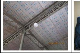
Factory did install the Manual Smoke Detector instead of interconnected smoke detection system N.C: Photo-01
